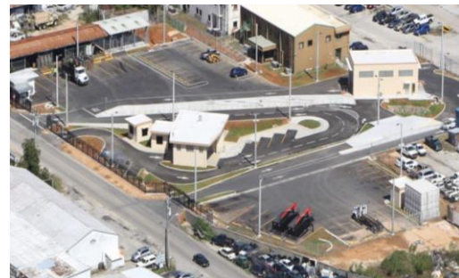
New Harmon Transfer Station and HHW facility
