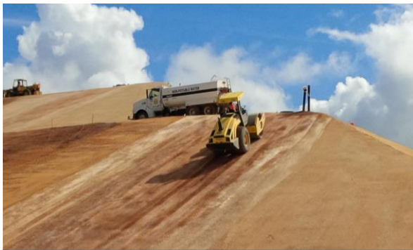
Soil cover foundation is compacted over Ordot Dump.
