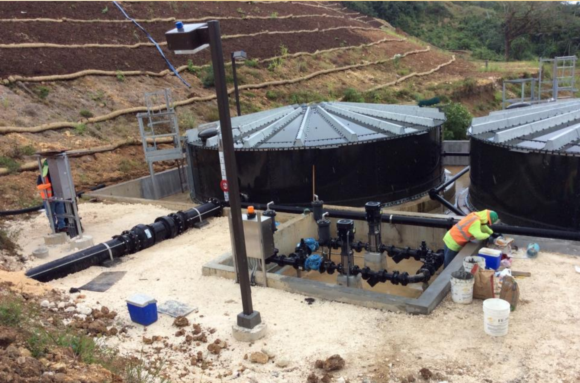
Leachate Storage Tanks and Pumps in Operation
