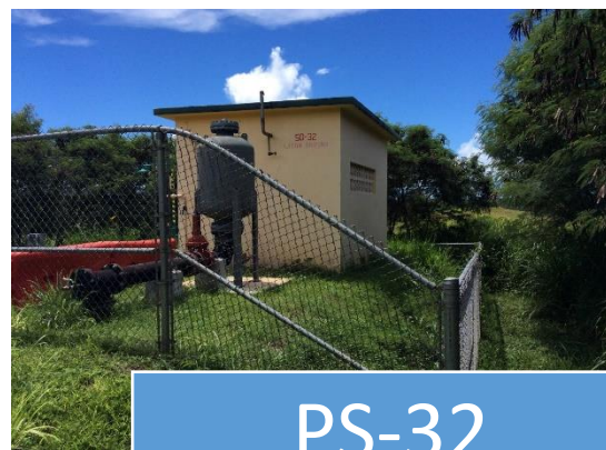
Figure 4 – Surge tanks installed at GWA pump stations
