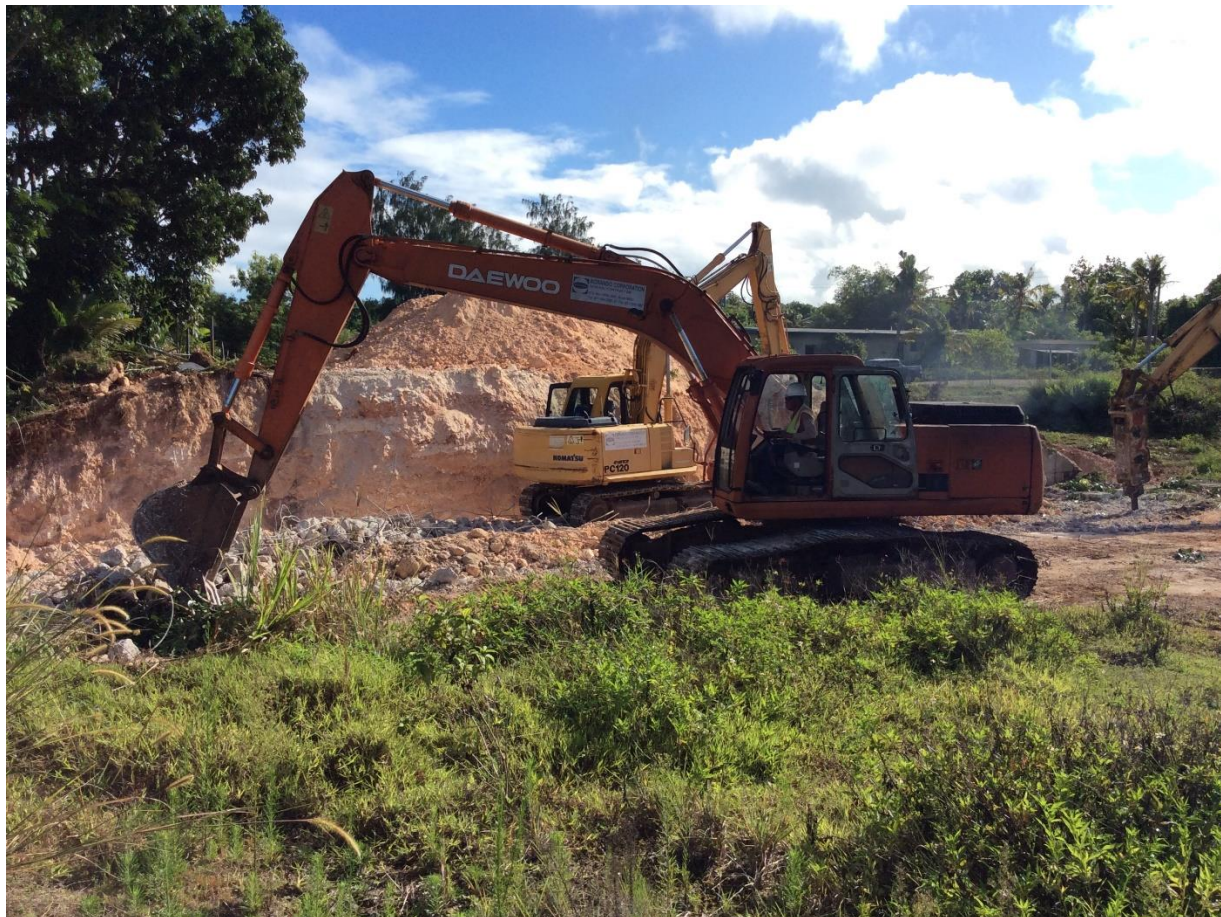
Figure 6 – Demolition of Dump Ramp at the Dededo Residential Transfer Station
