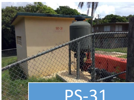
Figure 4 – Surge tanks installed at GWA pump stations
