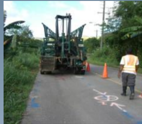
Drill rig setup
