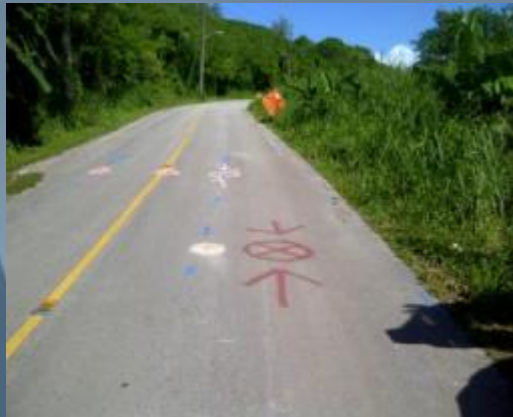
Dero Road drill location
